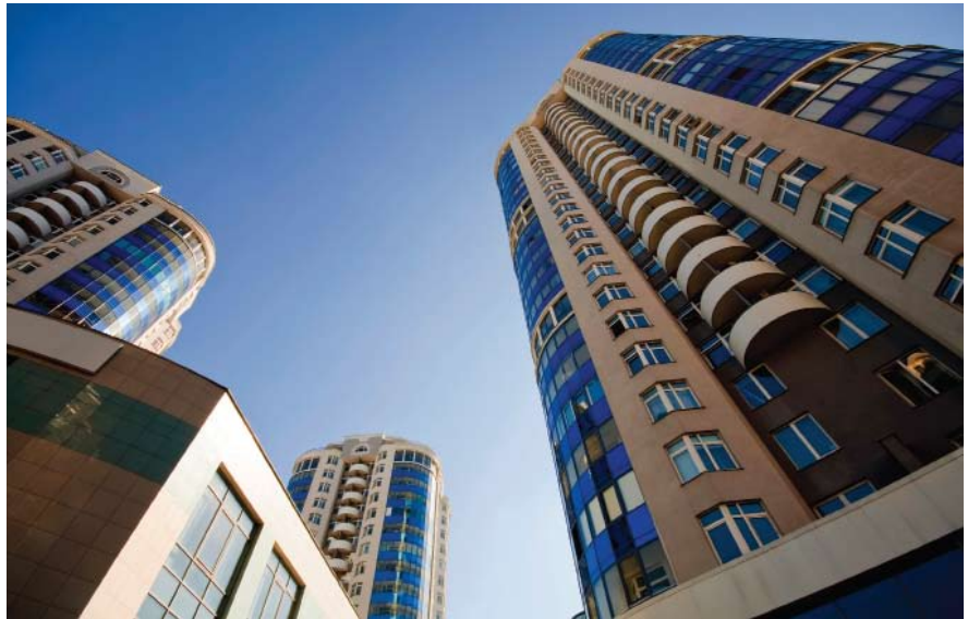
Modern apartment blocks are rapidly replacing the old Soviet-era ones in Ekaterinburg.
